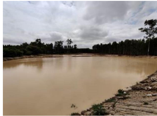
Nanjapura Lake after bottom dredging
